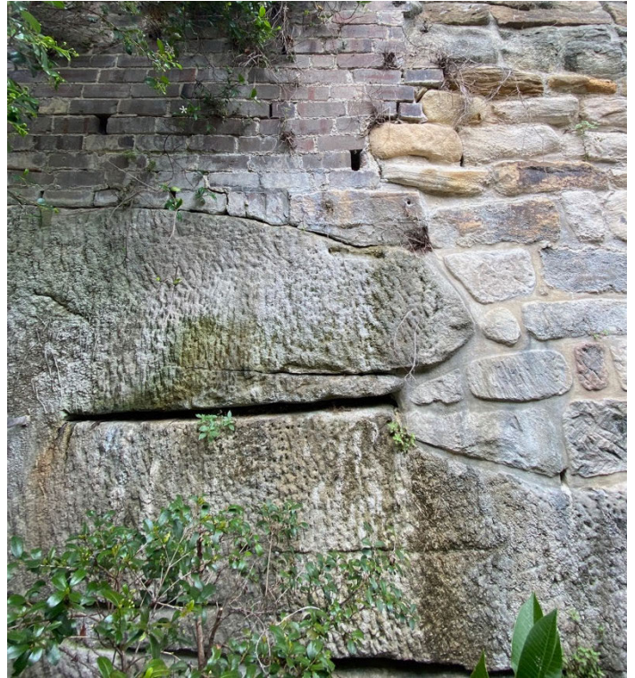
Retaining wall materials
