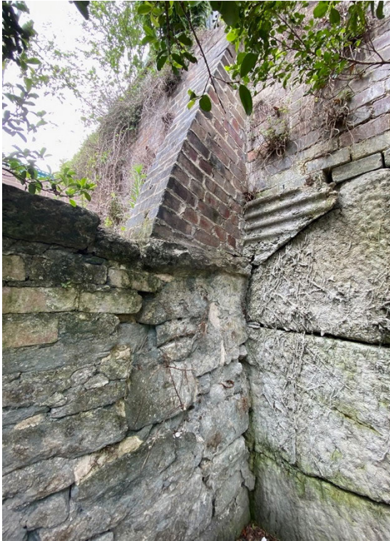
Brick buttress and retaining wall
